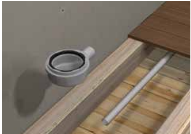
2. Install the waste ensuring adequate run off.
