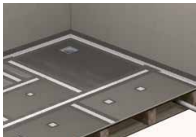
6. Seal all joints and fixings with waterproof joint sealing tape and corners. Your level access wetroom is now ready to tile.
